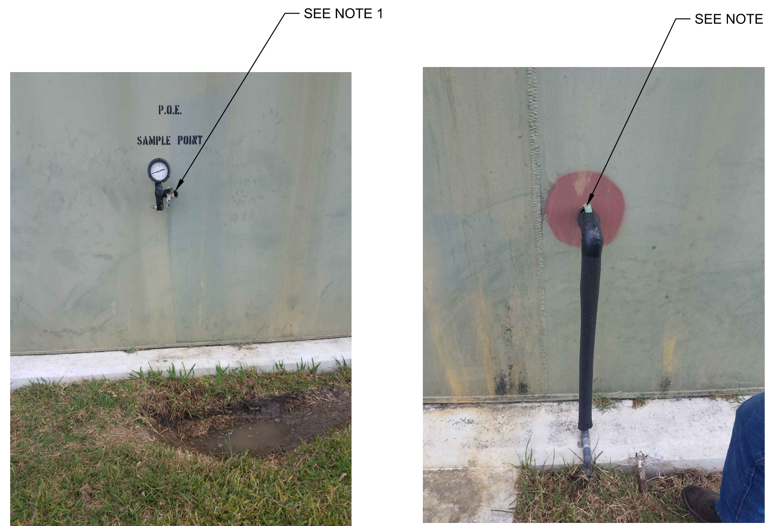
LOCAL SAMPLE PORT ONLINE ANALYZER SAMPLE PORT
